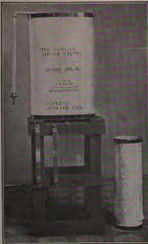
FIG. 60.— The Darnall filter, ready for operation.
